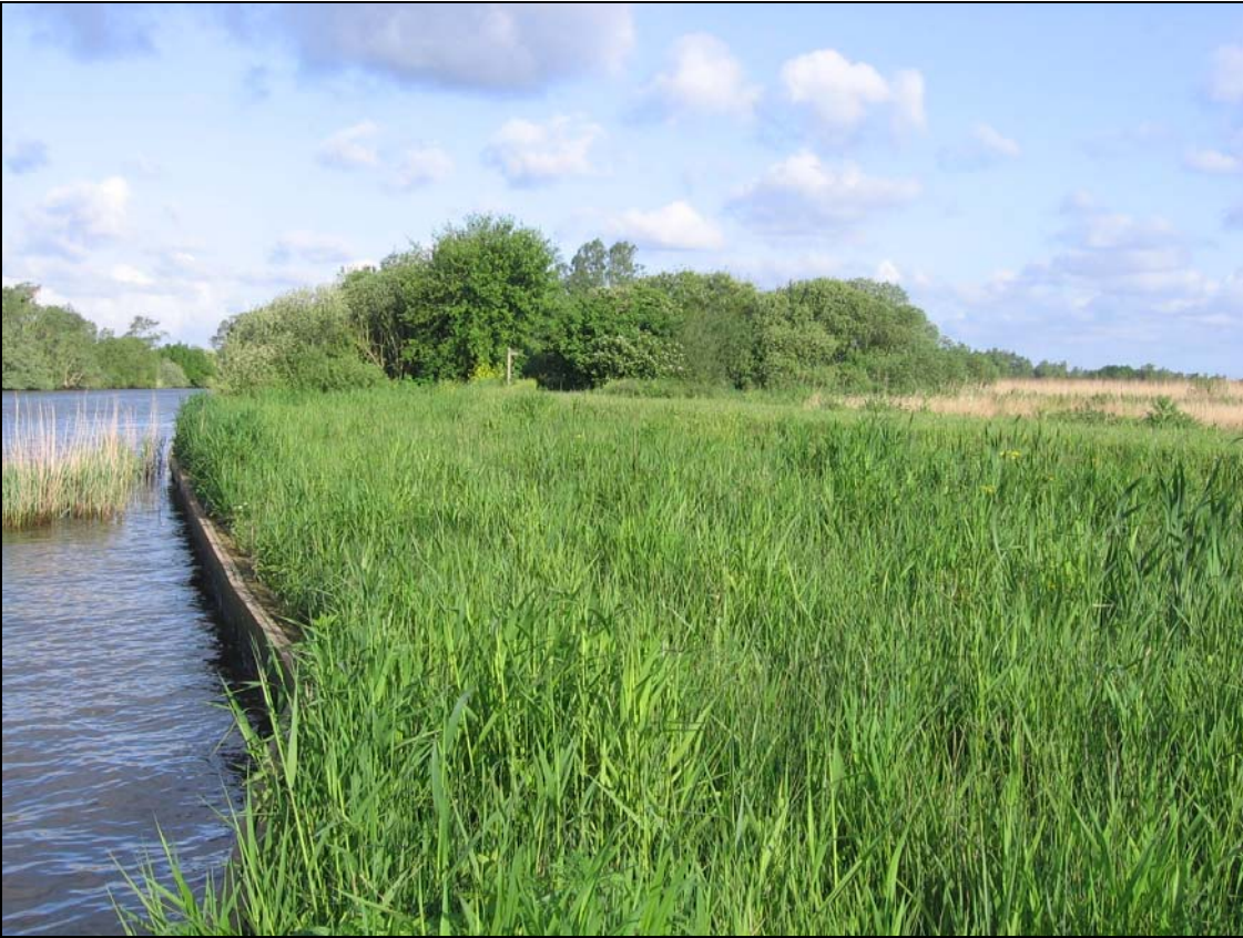
Newly established reed rond behind fence post piling, Strumpshaw
