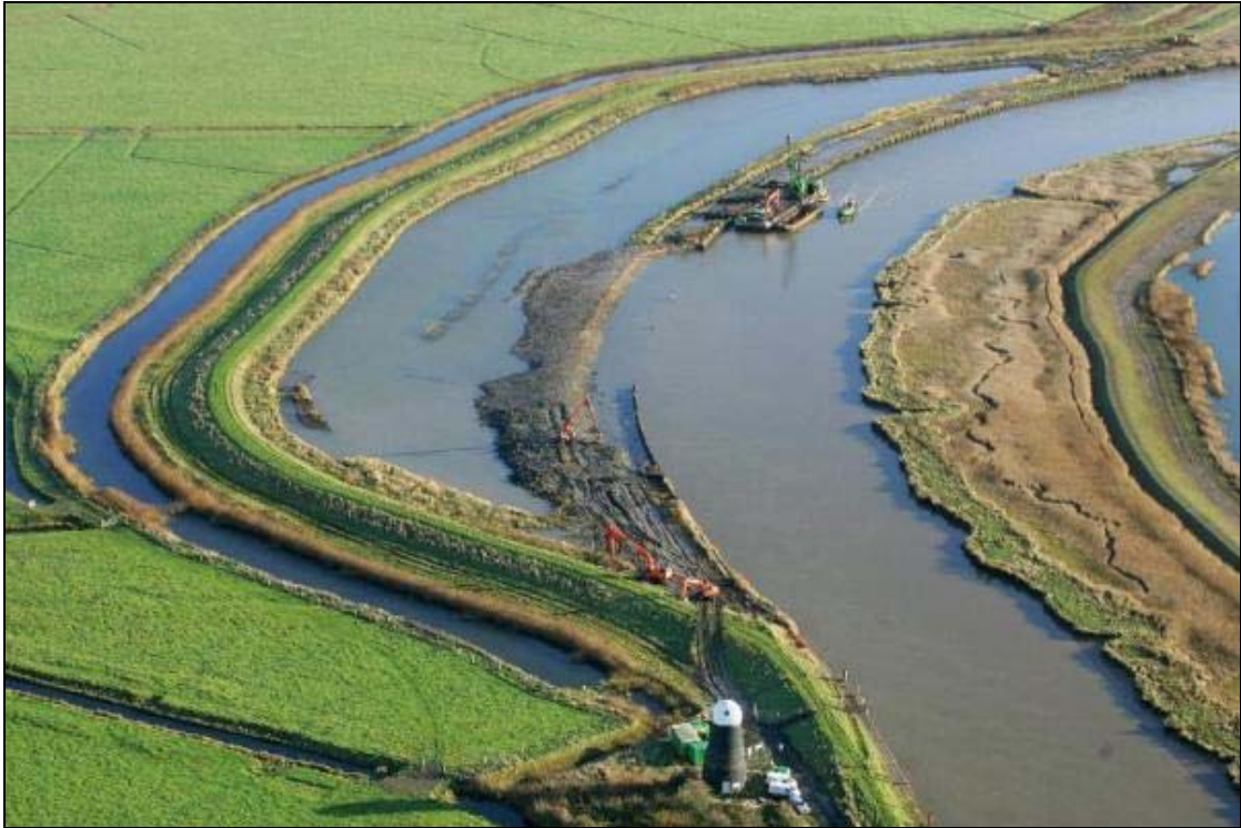
Setback bank & piling removal providing sustainable defences to protect the designated site and farming value at Halvergate (Photo: Mike Page)
